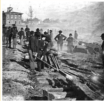
Dismantling Meridian's railroads. February 1863.
